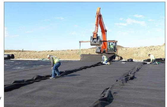
Workers lay the geotextile composite material on top of plastic liner.
