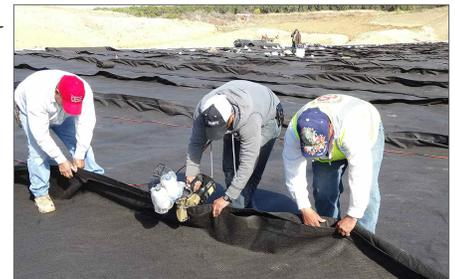
Workers sew the geotextile fabric together, which lays on top of the plastic liner.
