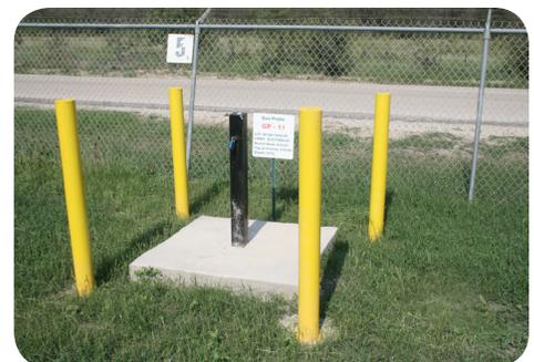
Gas probes, like the one above, are installed around the landfill. They are tested on a regular basis to determine if landfill gas is migrating off the site.
